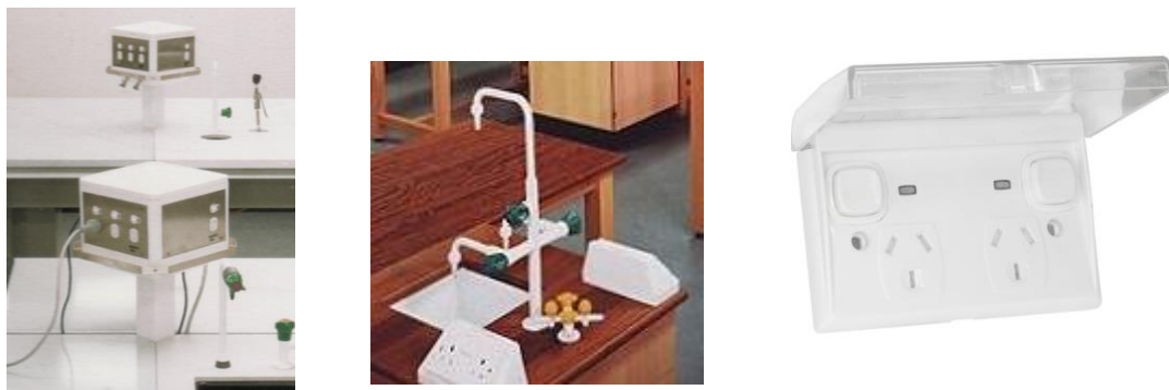
Figure 15: (L) An elevated service bollard, (C) a GPO orientated away from the water source, (R) a hooded GPO 54
