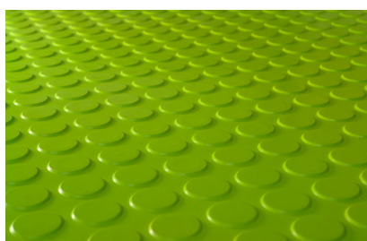
Figure 20: Sheet rubber with a high-relief texture is too uneven for trolleys and shoes with heels 75
